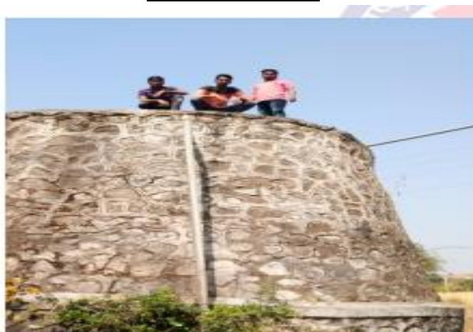
Water Tank Cleaning by NSS Volunteers Dated 14/02/2019
