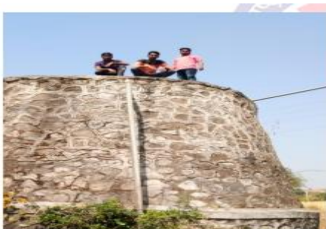
Water Tank Cleaning in Ghogaon village dated 14/02/2019
